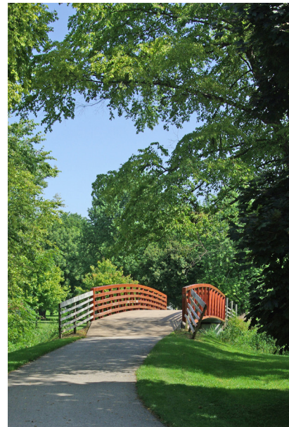
Washington Street bicycle route connects to a pedestrian bridge in Marquette Park
